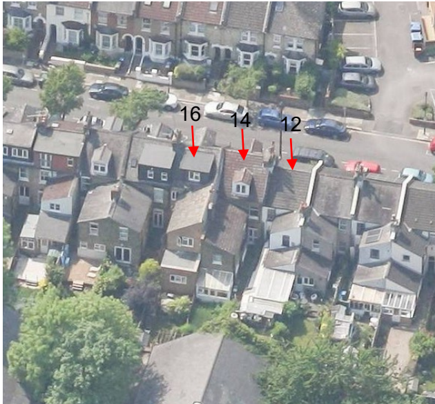
Image 1: Rear building line of relevant section of Shirley Road.
